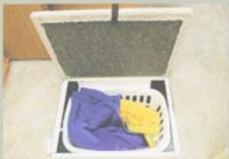
An in-floor laundry chute and basket cleverly conceals soiled laundry underneath the floor.
